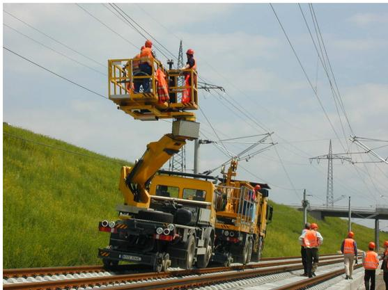
Fig. 5: Bearer cable for overhead line
