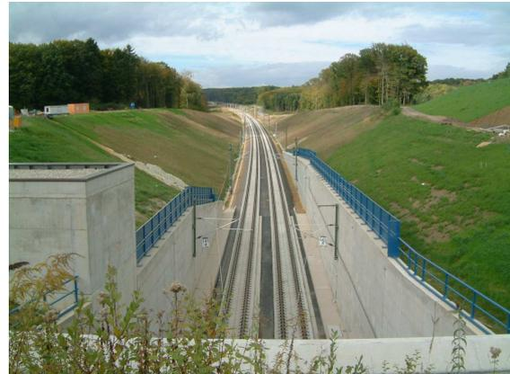
Fig. 2: Overhead line at the northern portal of the Schulwald tunnel
